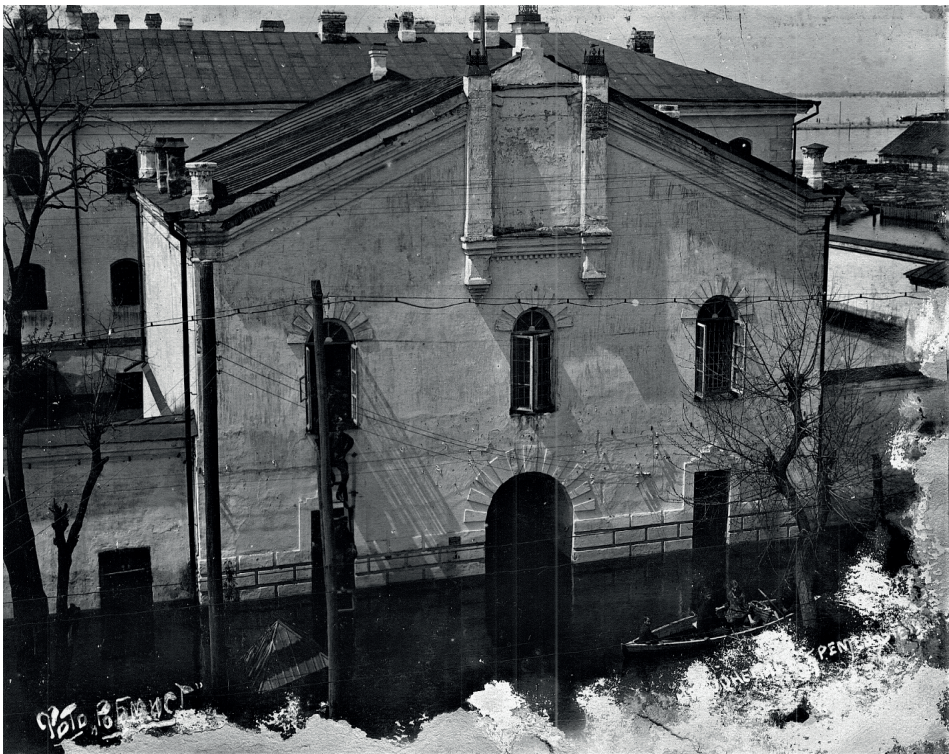
Figure 1 – Former prison gate church «Joy to All Who Sorrow» 1931.
